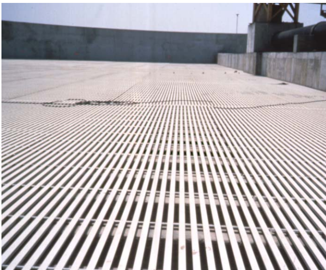
Above: Fiberglass grating was installed as media trickling filters at the Des Moines, Iowa Wastewater Treatment Plant.
