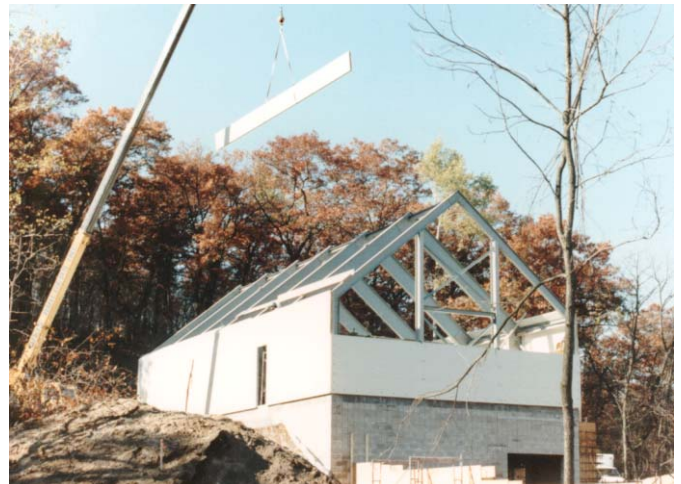
This all-fiberglass facility for Amador Corp. assures RFI/EMI compliance in testing computers as well as other manufactured equipment.
