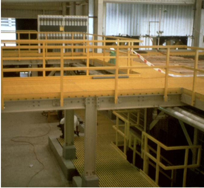
Above: Fiberglass walkways and operating platforms are used extensively in the highly corrosive SXEW copper refinery at Minera Escondida Limitada, Chile.
