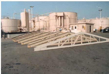
Above: Trusses for this tank cover used at a Shell Oil Refinery were preassembled and shipped to the site...
