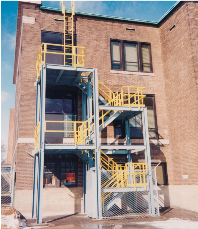
Above: FRP was chosen for this three-story fire escape because fiberglass would not require painting or maintenance.
