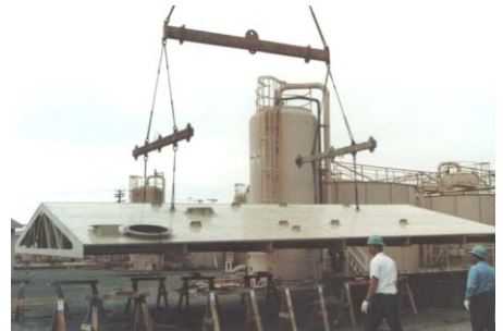
... final fabrication using EXTREN® plate and fittings was easily completed at the site.
