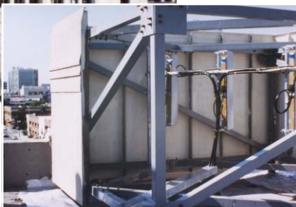
This all-fiberglass facility for Amador Corp. assures RFI/EMI compliance in testing computers as well as other manufactured equipment.
