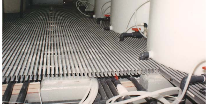
Above: A raised floor, in the processing room of a California film development laboratory, surrounds existing equipment, provides access above and below the floor, withstands the corrosive environment and provides 200 lbs/sq.ft. load capacity to support heavy machinery.
