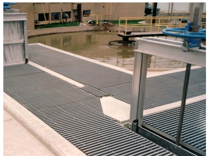
Above: Low maintenance fiberglass grating provides trouble free operations for the Wastewater Treatment Plant Headworks covers and walkways in Lakewood, Colorado.
