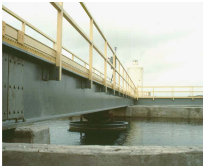
Above: Lightweight, corrosion resistant 24" fiberglass I-beams span 45' to bridge clarifiers at the Las Rusias, Texas Waste Water Treatment Plant.
