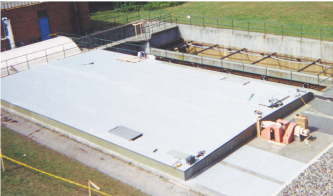
Odor control covers at a wastewater treatment plant in Smithfield, Rhode Island, will withstand the corrosive environment to provide years of trouble-free service.
