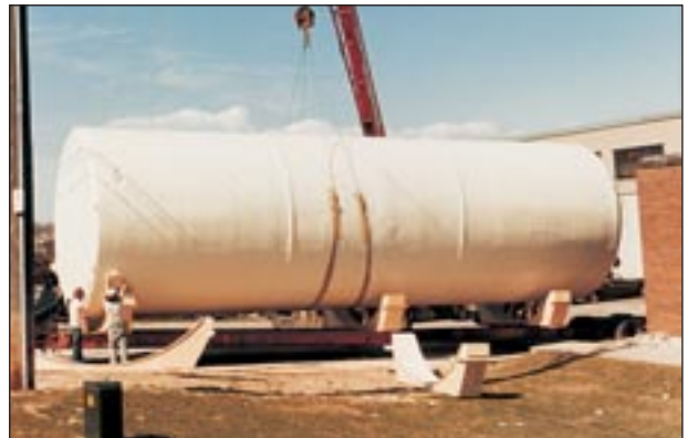
FOOD INDUSTRY: ▶ 12' Diameter / 35' High 14 Tanks Insulated — Steam treated
