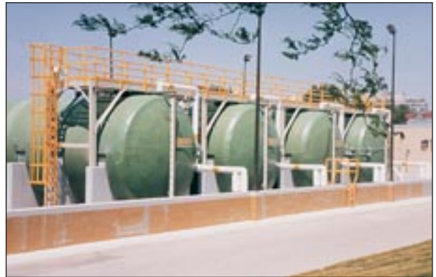
ALUM WATER TREATMENT: ▶ 13'6" Diameter / 30' Long 4 Tanks Heat traced — Insulated — Horizontal
