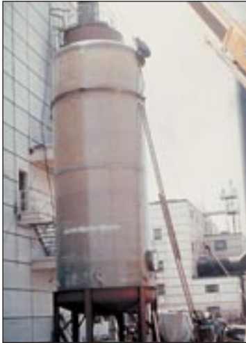
◀ NICKEL CHLORIDE SLURRY: 12' Diameter / 33' High 20 Tanks for high sp. gr. slurries
